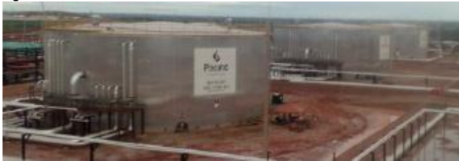
Figura 8. Free Water Knockout CPF-2
